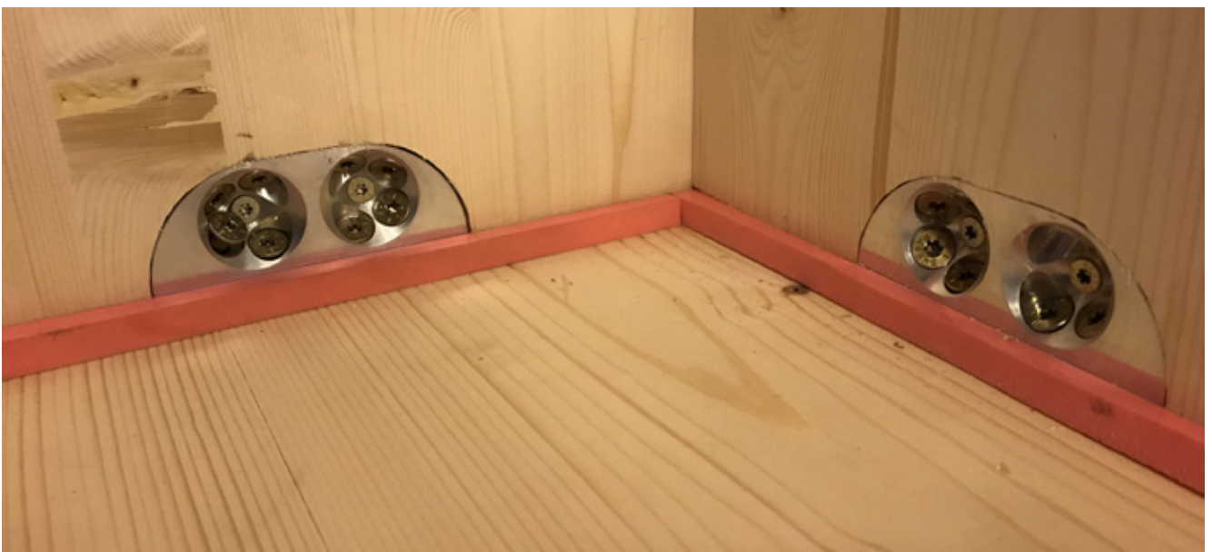
Fixing with SHERPA CLT connector
