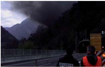
Figure 6.8: Tunnel fire test 2001 in a Brenner Motorway tunnel in cooperation with the Autostrada del Brennero S.P.A. Institute for Constructive Civil Engineering, Santa Automation Instruments and fischer fixing systems [1]
